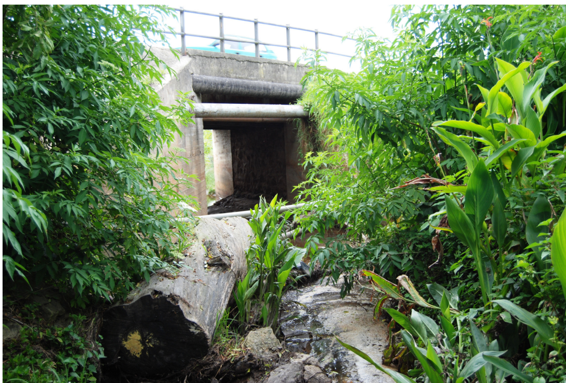
Wellington Street Bridge looking down stream. Notice service lines obstructing debris.
