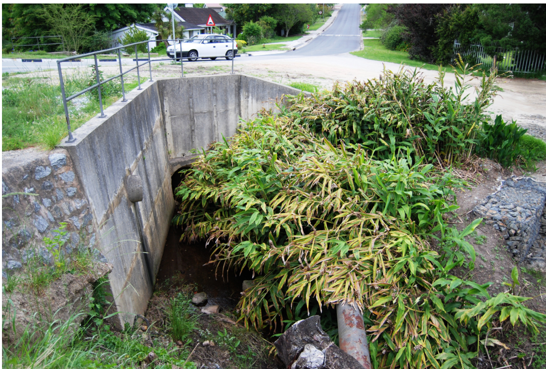
Adderley Street Bridge looking down stream. Notice exposed service line causing obstruction.
