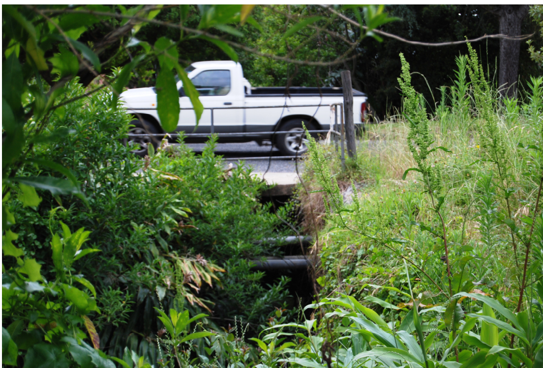
Kerk Street Bridge looking down stream. Notice exposed service lines.
